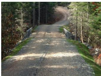
Photo: Lefort Road Bridge, Cape Breton, PHP
