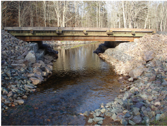
New bridge installation, Paul MacDonald, PHP
